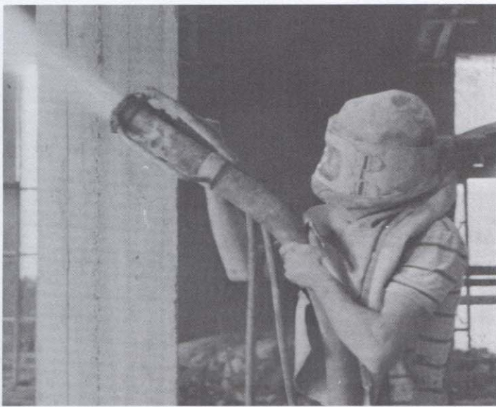
INNOVATION CARRIES OVER TO THE RECONSTRUCTION OF PRINCETON HALL, WHERE AN ASTRONAUT-LIKE MASON APPLIES GUNITE (A MIXTURE OF SAND AND CEMENT), USING A HIGH-PRESSURE CEMENT GUN, ADDING TENSILE AND COMPRESSION STRENGTH TO THE FARM SCHOOL'S "PARTHENON" AS EARTHQUAKE PROTECTION.
