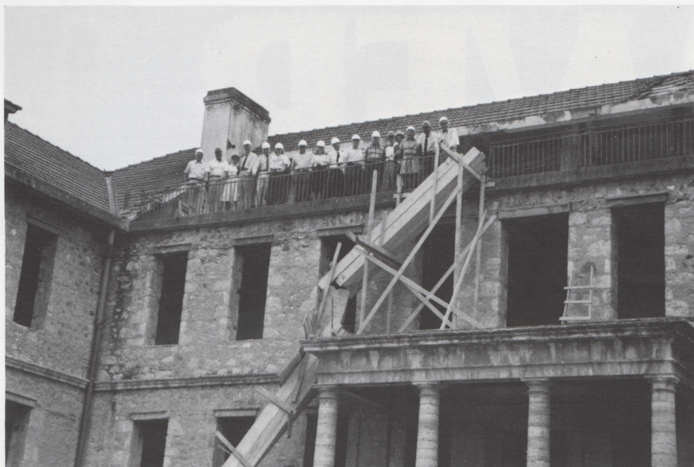
Trustees inspect Princeton Hall renovation in May, 1984.
