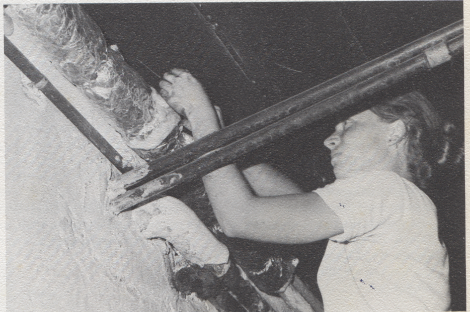
Maria Applewhite helps the Farm School save energy by installing insulation.
